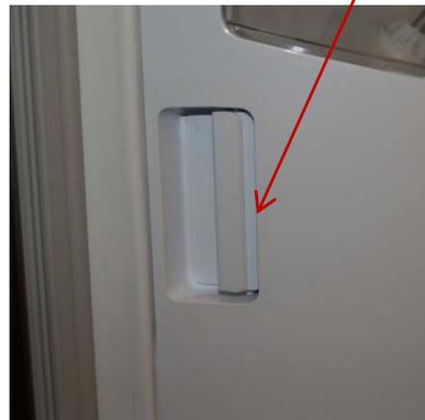
Ice bucket reed switch, Ice Off LED flashes if bucket is not in place
